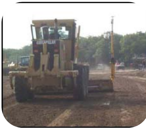
3D Control of Subsurface Preparation
