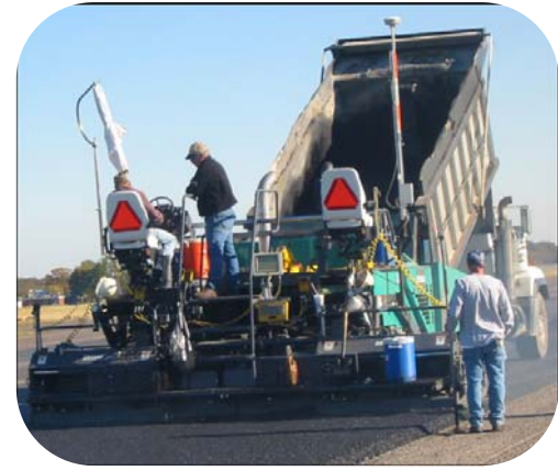
GPS/RTK System Controls Paver Movement
